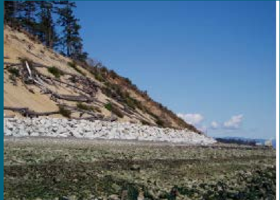
Sediment supply reduced after installing riprap protection
